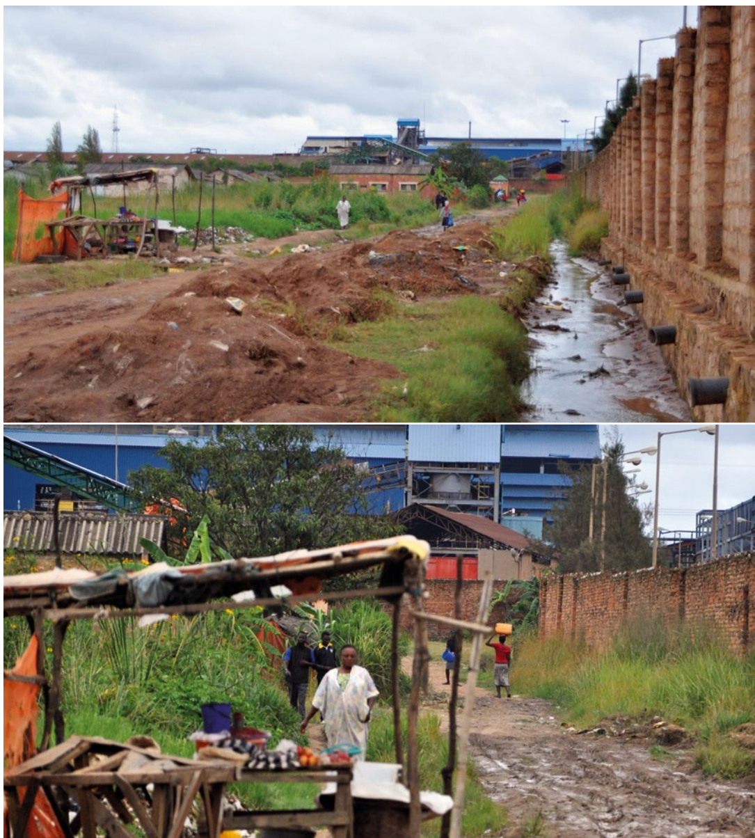
Communities living next to Chemaf's plants have serious concerns about air and water pollution. The pictures show one public road adjacent to the wall of the Chemaf property. The upper picture includes Chemaf drainage systems connecting to the public sewage system. The blue buildings in the back are Chemaf's. 65
